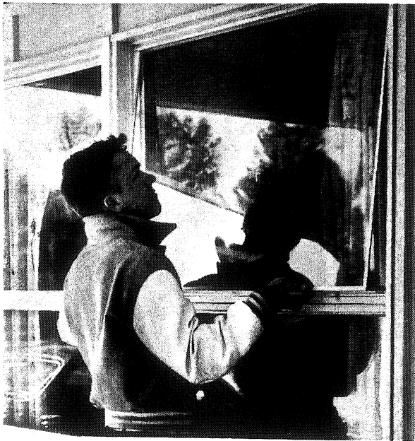
Fig. 2 Installation of third pane of glass
