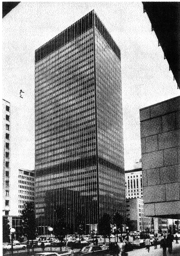
FIGURE 3. Thirty-four-story office building looking southeast (relative to building). Dark bands are at 10th and 33d floors, where mechanical services are located and wind pressure measurements were taken.
