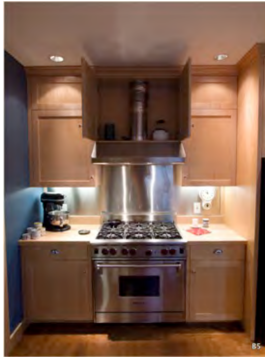
Figure 55. Exhaust System B5; placement in kitchen.
