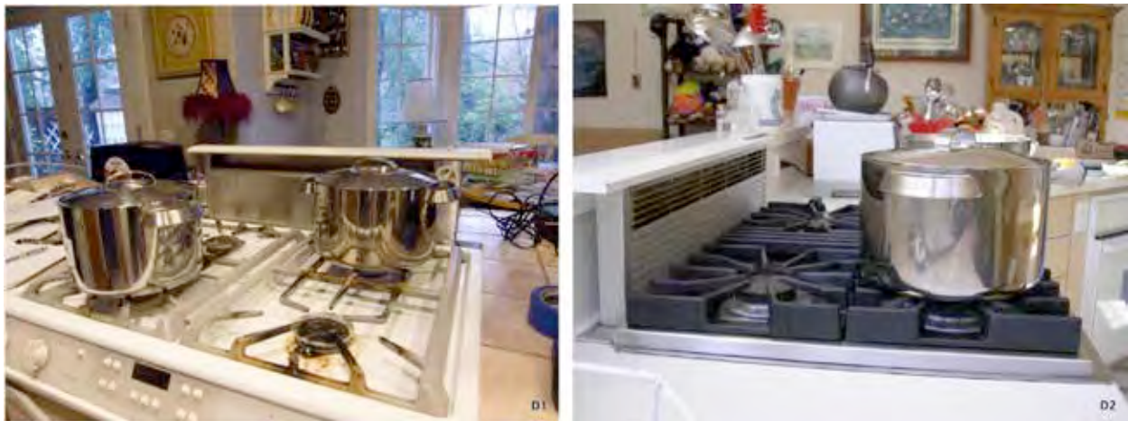
Figure 2. Rear downdraft exhaust systems D1 and D2
