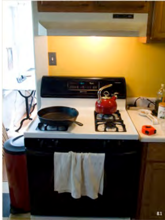
Figure 39. Exhaust System B1; note hallway at left.
