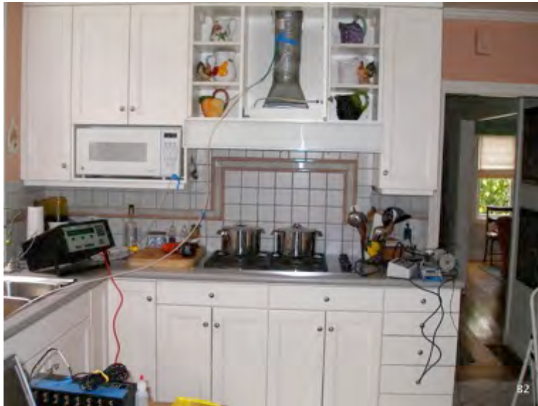
Figure 43. Exhaust System B2; placement in kitchen.
