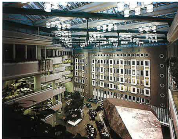
Picture 24 Hall Seen from Upper Floor
