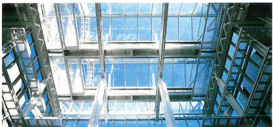
Picture 36 Roof Construction
