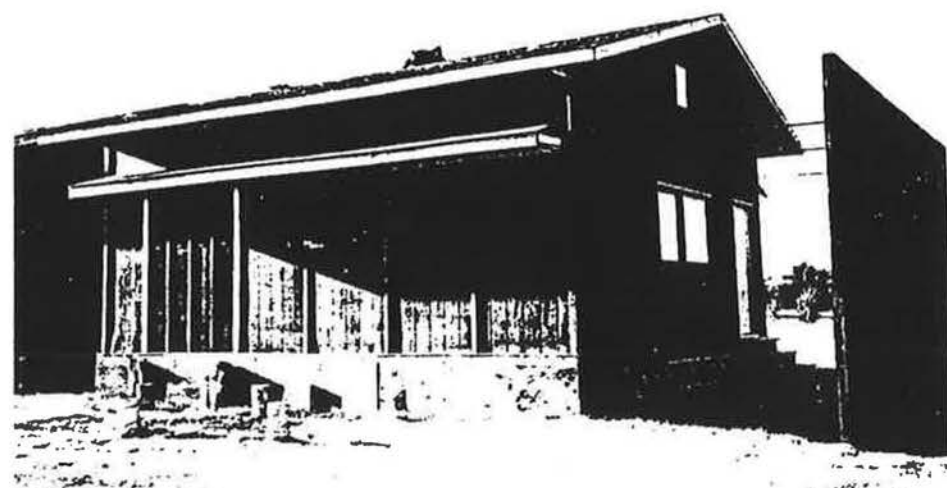
Figure 5-1. Houses 5 and 6 at AHHRF showing building orientation and false end wall.
