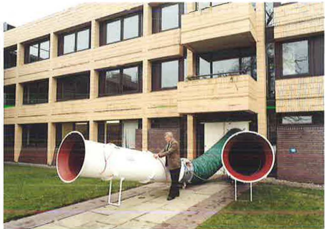
Pressure testing a whole building
