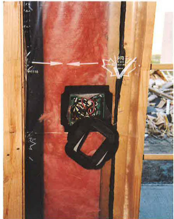
Special electrical services seal, as used in Canada. Similar seals are now available in the UK
