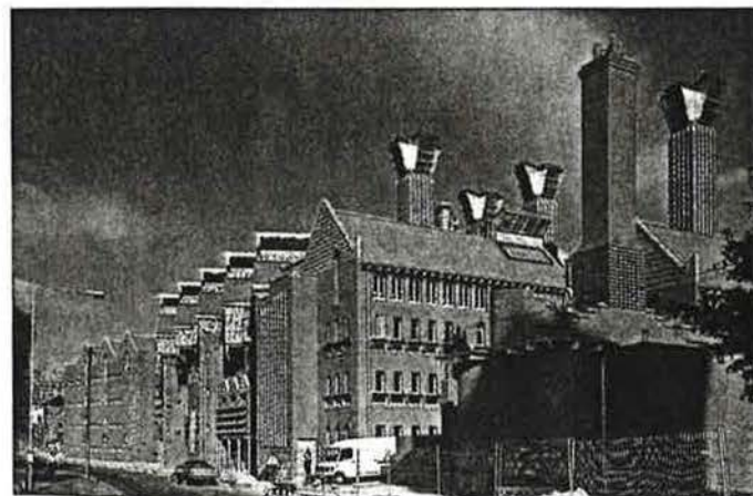
The NW elevation facing Mill Lane. Note the natural ventilation stacks and glazed ventilators in the roof gables.
