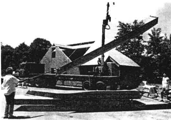
Figure 4 Roof components being installed on the proof-of-concept structure.
