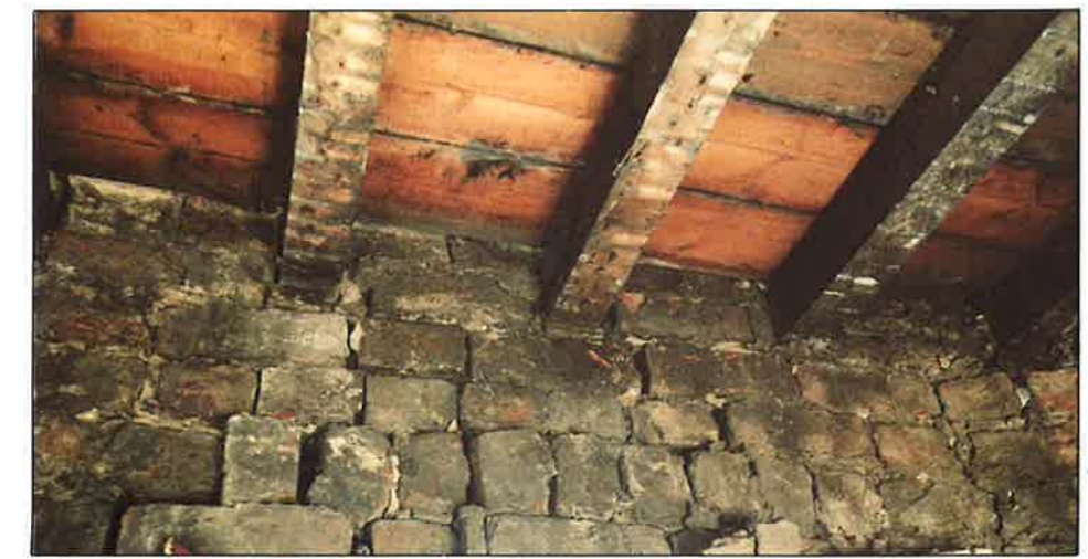
Figure 2. Decaying timbers
