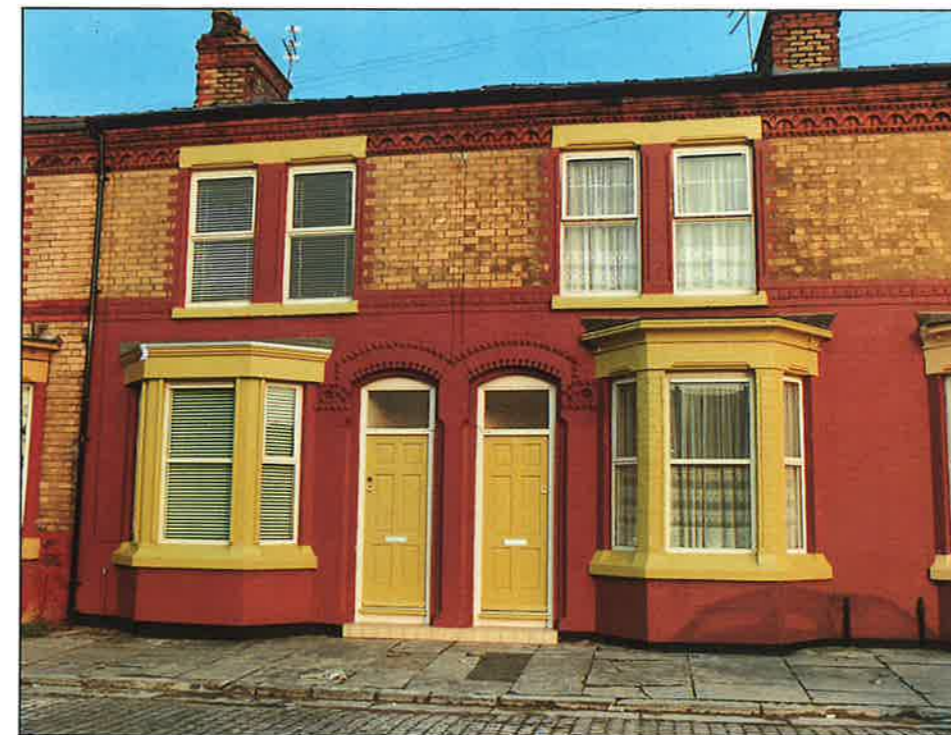
Figure 1. Refurbished Pre 1919 houses on Merseyside
