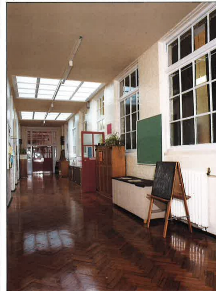
Examples of where an insulated suspended ceiling is, and is not, appropriate. The top floor corridor at Hither Green School is the former, while the top floor hall is the latter
