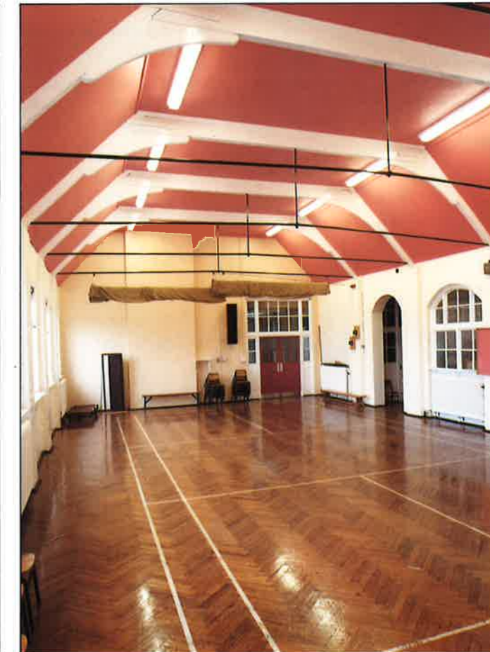
Examples of where an insulated suspended ceiling is, and is not, appropriate. The top floor corridor at Hither Green School is the former, while the top floor hall is the latter
