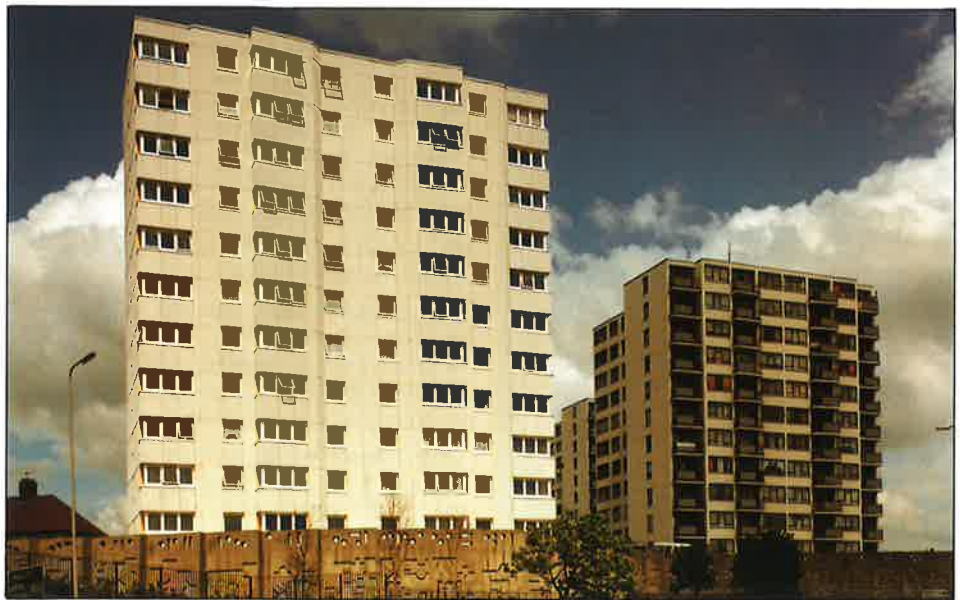
Knowsley Heights – refurbished block on the left of picture
