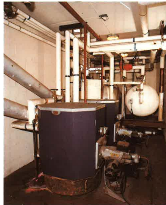
The original heating plant (left) at Holly Court and (right) new condensing boilers
