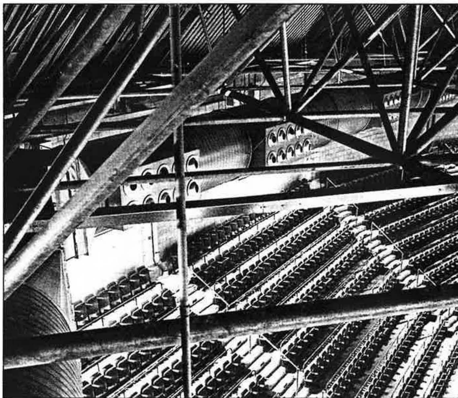
Air is blown at high level via nozzle diffusers in this sports arena.
