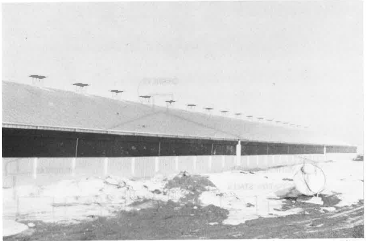
Photo 3. Naturally ventilated breeding-gestation unit with insulated vertical sidewall panels complete with windbreaks and intermittent chimneys.
