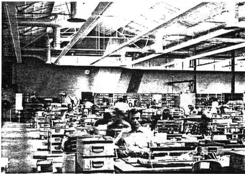
Fig. 5. An industrial hall with a turbulent air supply
