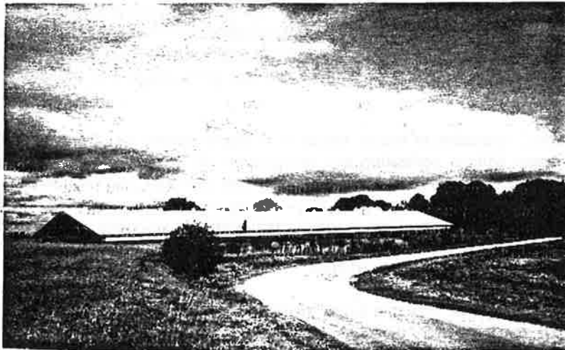
Fig. 1. Photo of the broiler house seen from south-west.
