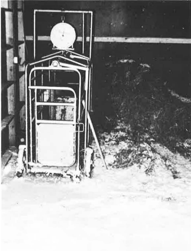
Fig 3 Snow which had penetrated a capped open ridge lying within a building
