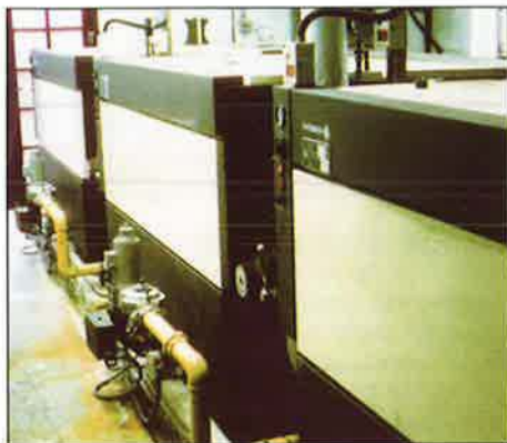
Trowbridge County Hall boiler house
