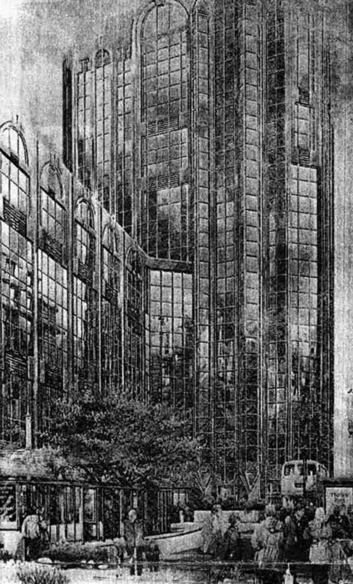
The Colmore Gate development in Birmingham will have high frequency lighting and low level perimeter heating to limit SBS.
