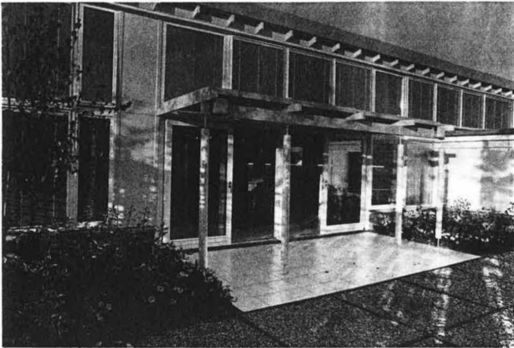
Figure 1 View of superglazed house from courtyard
