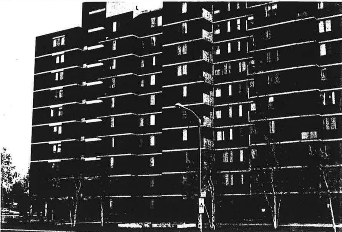
In Toronto, a 10 storey condominium building was selected for the project. This building is also heated with electric baseboards but the corridor make-up air is heated with natural gas.
