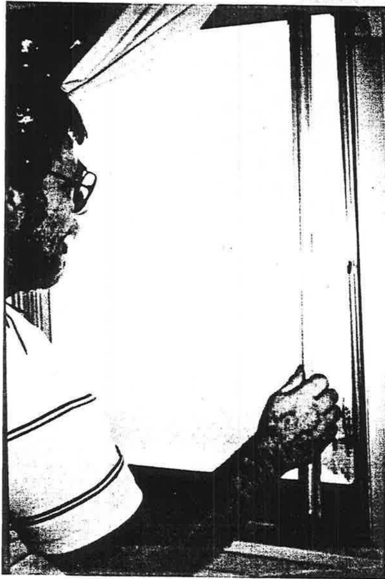
Window sashes were removed, the weatherstripping was replaced then the sashes were reinstalled.
