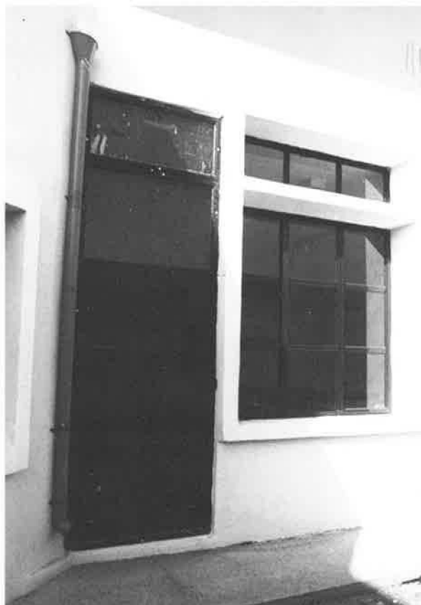
Figure 17. Detail of Trombe wall
