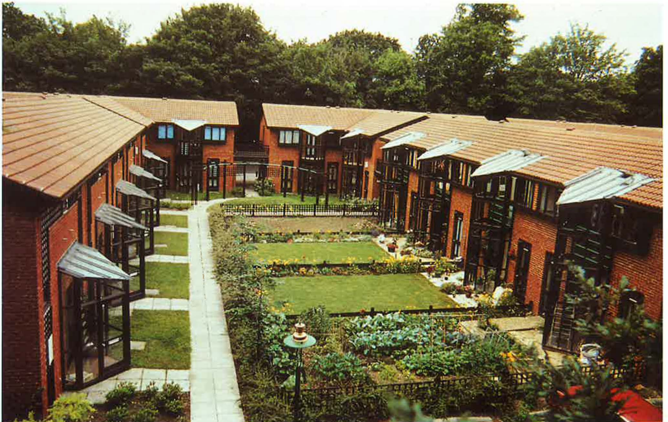
Fig 25 Spinney Gardens housing; view looking NW. Courtesy of PCKO Partnership and ETSU
