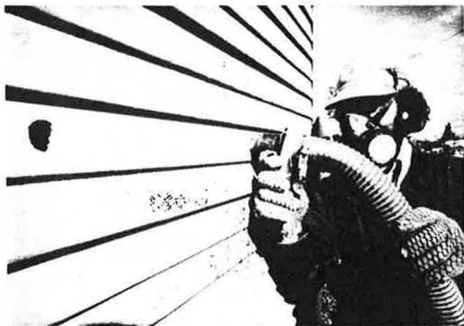
Effective, inexpensive, and environmentally benign, blown-in cellulose is a popular insulation material, and reduces air leakage in walls.
