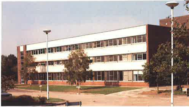
Figure 3 Southwest elevation of office building
