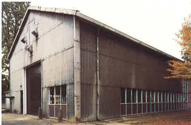
Figure 4 North elevation (door) of hangar building
