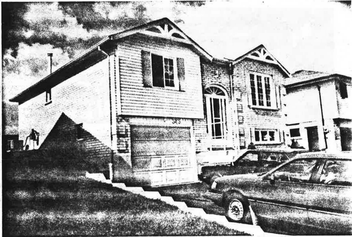
Photo 1 - House in Guelph Ontario With a Hard Connected Fresh Air Duct Connected to the Return Air System
