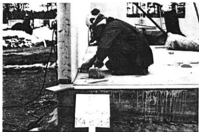
Fig. 10. A wall element is placed on the steel sill
