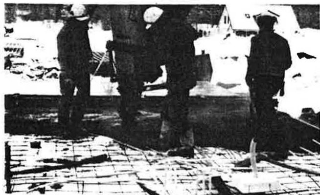
Fig. 2. Casting the concrete slab (March 1985)
