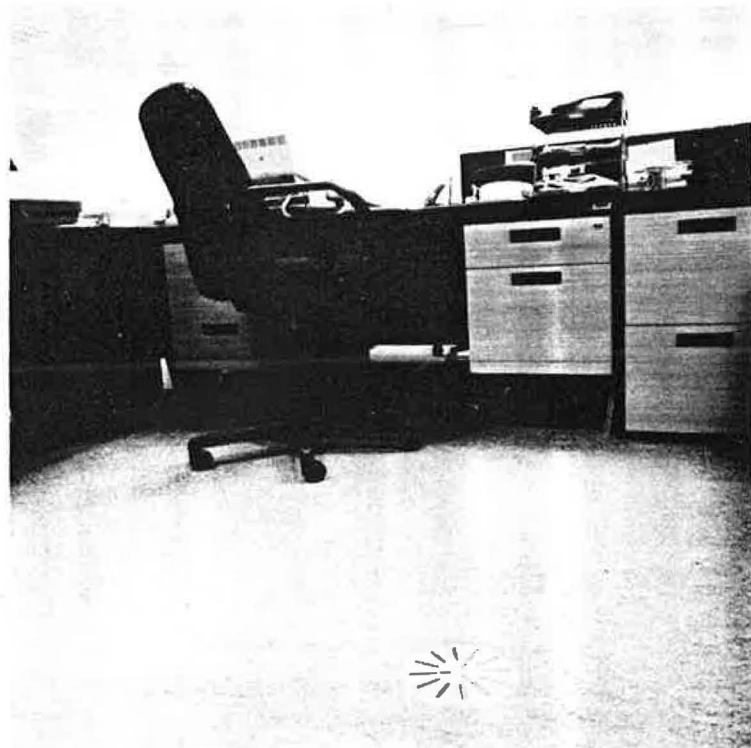
Fig. 3. Air supply terminal in floor
