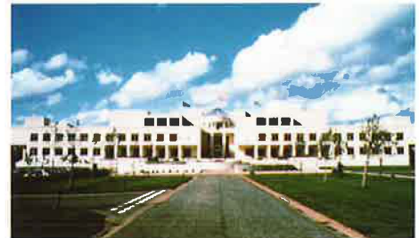
NFU Mutual and Avon Group Head Office designed to avoid air conditioning in most areas
