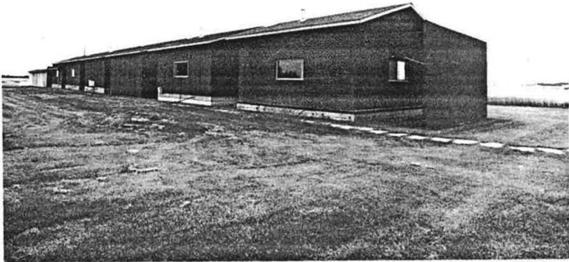
Figure 3-1 North side of test houses looking east along row from Masonry Unit 1 showing rain-capped flues and end wall wind shielding barrier.
