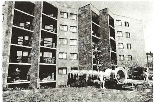
Figure 1 Test building showing test setup for measuring airtightness of the building envelope
