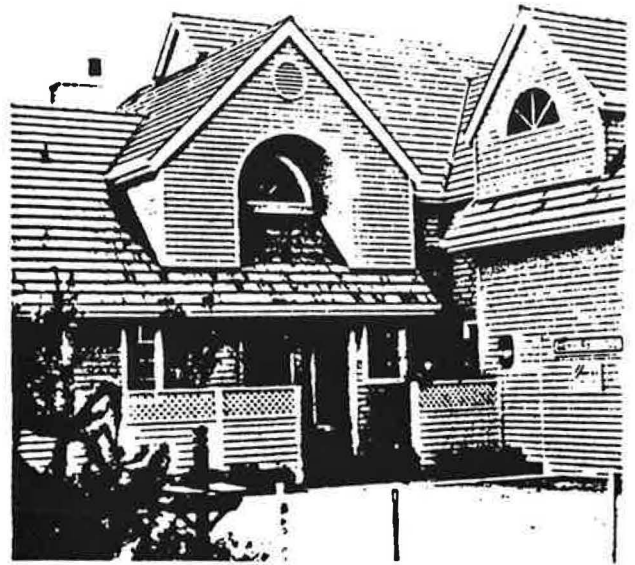
The objective of the study is to identify the average ventilation rate for homes constructed in the Northwest region since 1980.
