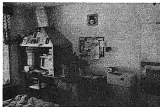
Figure 1 An extreme example of remedial action taken: a special fume hood to remove emissions given off by computer, VCR and TV.
