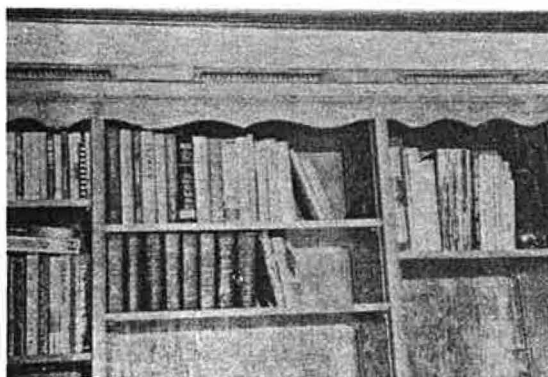
Figure 2 Even books can give off emissions. Exhaust grilles over book case.
