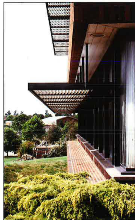
Typical office windows with overhangs and sunscreens.
