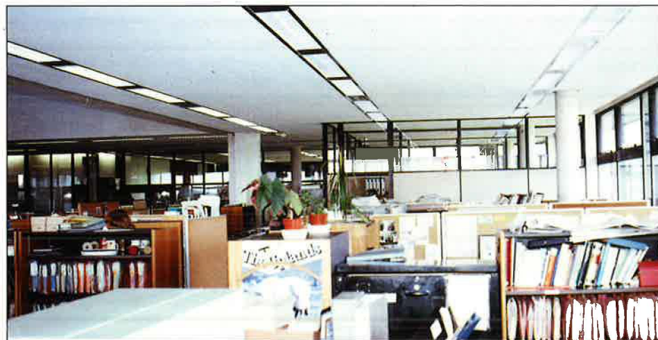
Perimeter offices. Note that the band of lights towards the window is off under automatic control.
