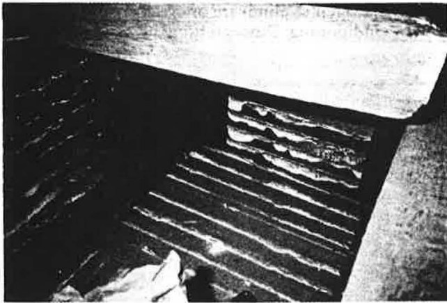
Looking down from the attic into the top of a drop-ceiling closet. Notice the stud-bay bypasses.
