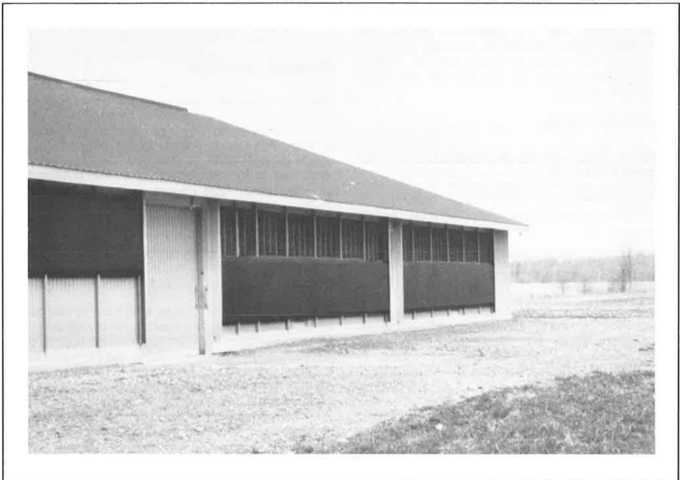
Insulated vertical panels are shown in both the open and closed positions on a turkey barn.
