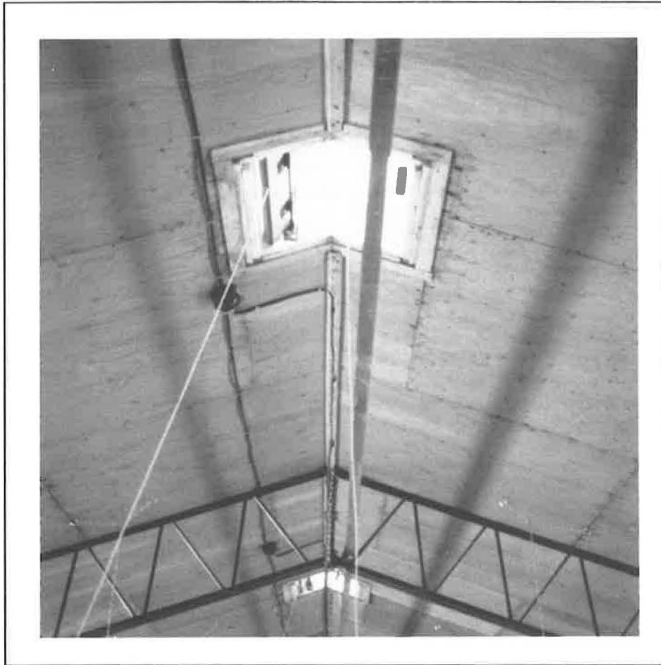
Chimneys with baffle and manual control cable as seen from below. The baffle is in the fully open (summer) position.
