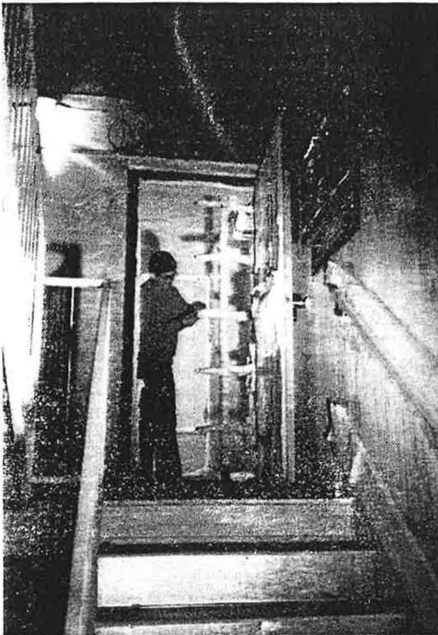
Figure 3 Velocity pressure tubes at open stair door
