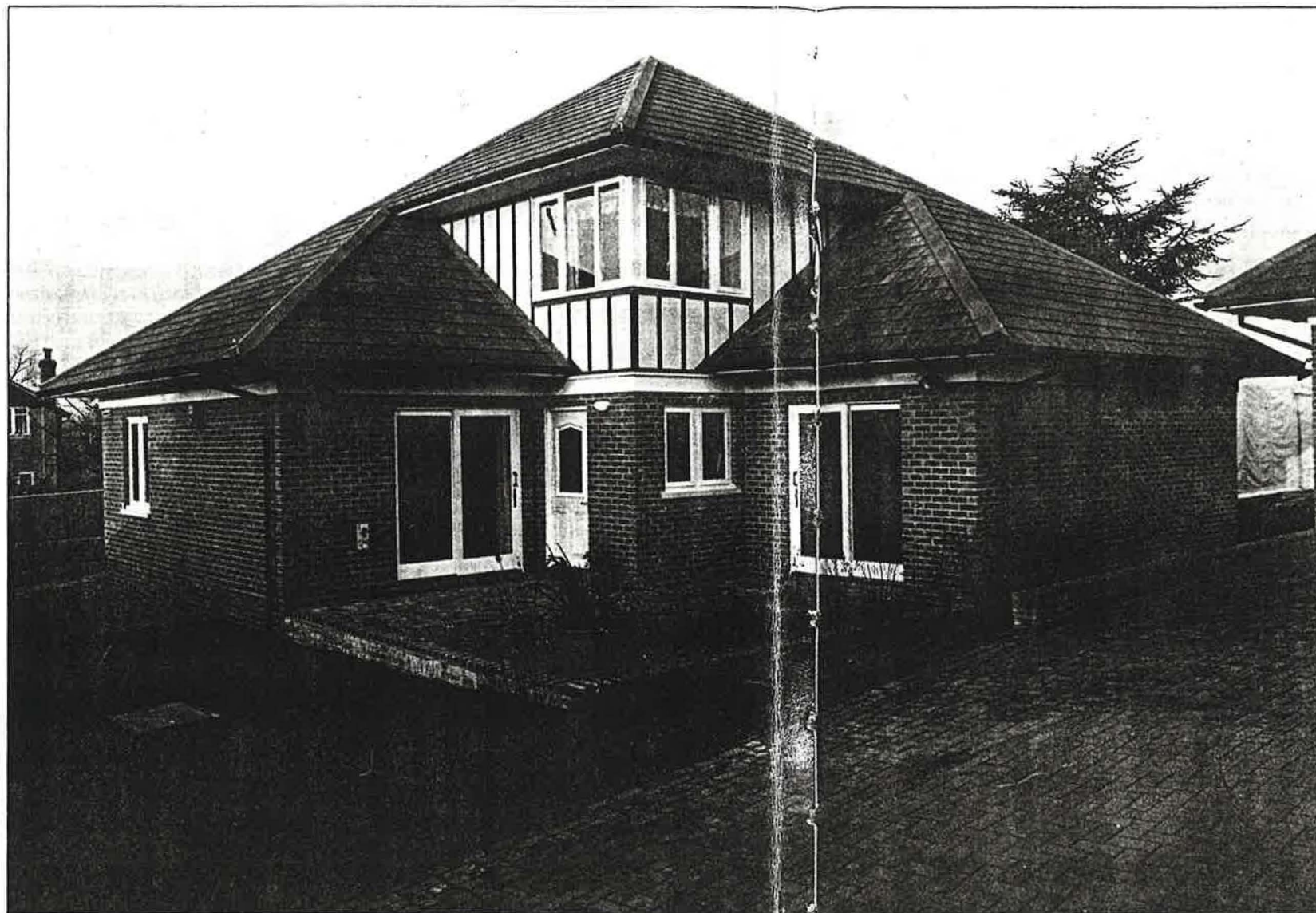
Energy management control guided the design of this prototype bungalow
