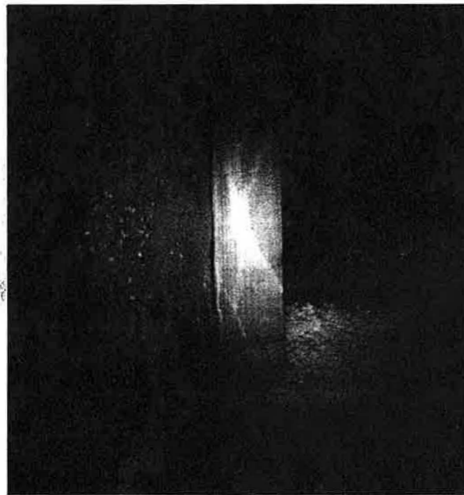
Above: Missing insulation in a wall cavity. The concept of electric heating in buildings reinforces the need for good quality control during construction.
