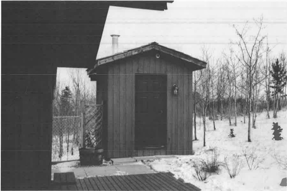
ISOLATED BOILER ROOM
