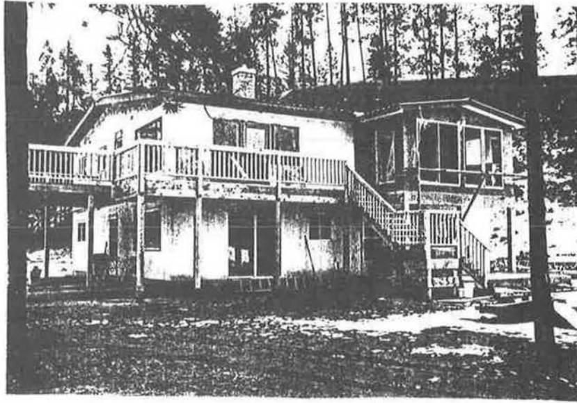
EXTERIOR VIEW SHOWING ADDITION UNDER CONSTRUCTION
