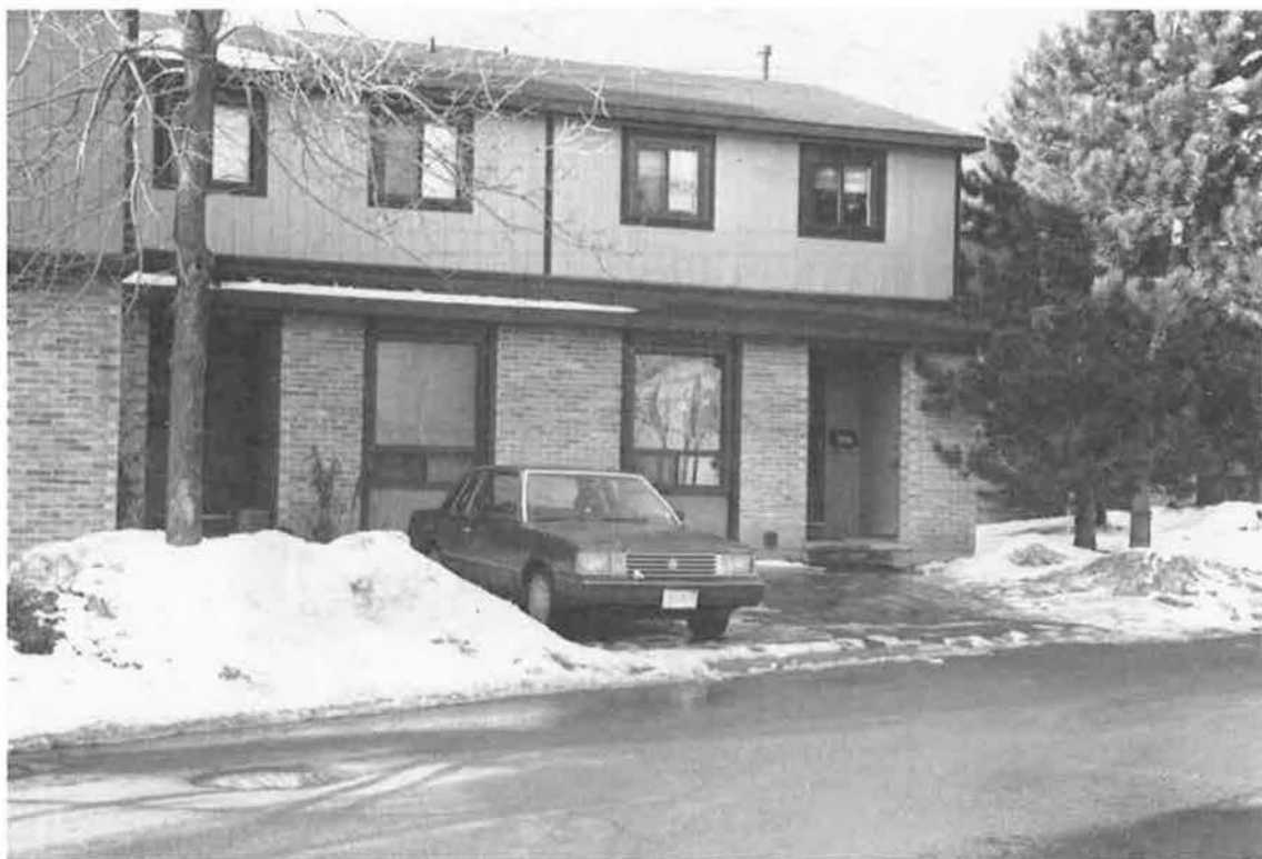
EXTERIOR VIEW TOWNHOUSE UNIT
