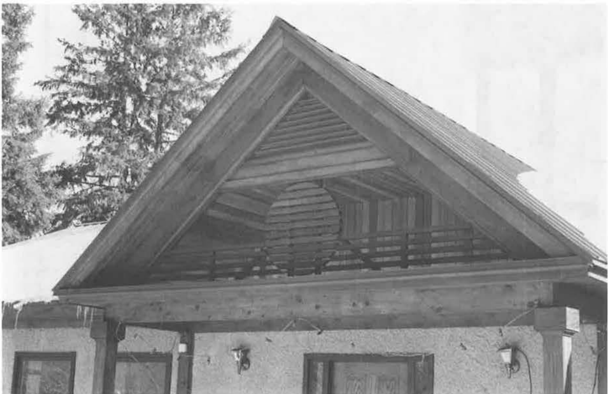
EXTERIOR DETAIL, SHOWING AIR INTAKE IN GABLE END
