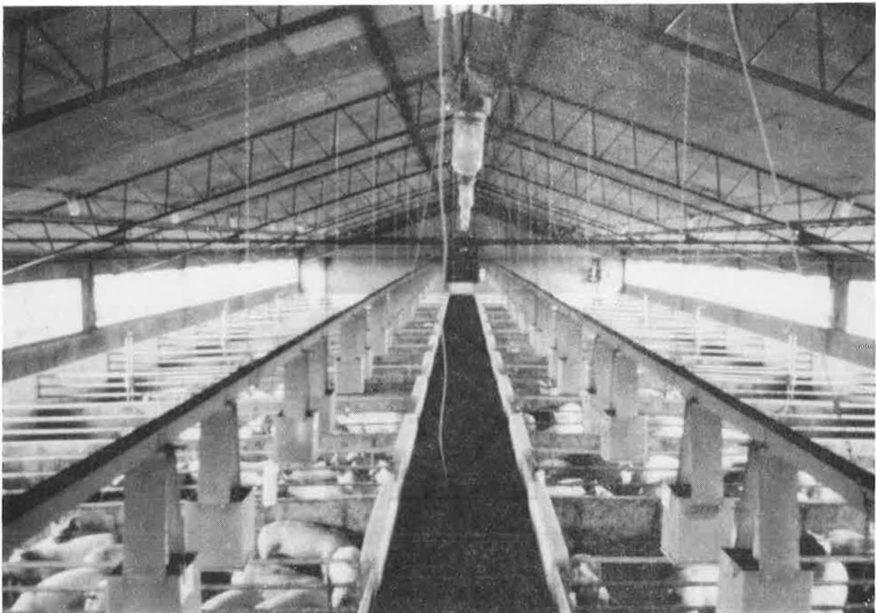
Photo 2 Natural ventilation will provide an excellent environment in this warm insulated steel-truss building with a sloped ceiling.
