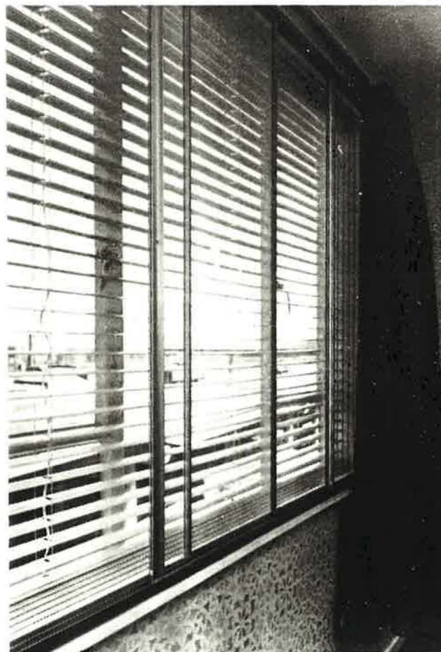
Figure 1 Secondary double windows with mid-pane venetian blinds
