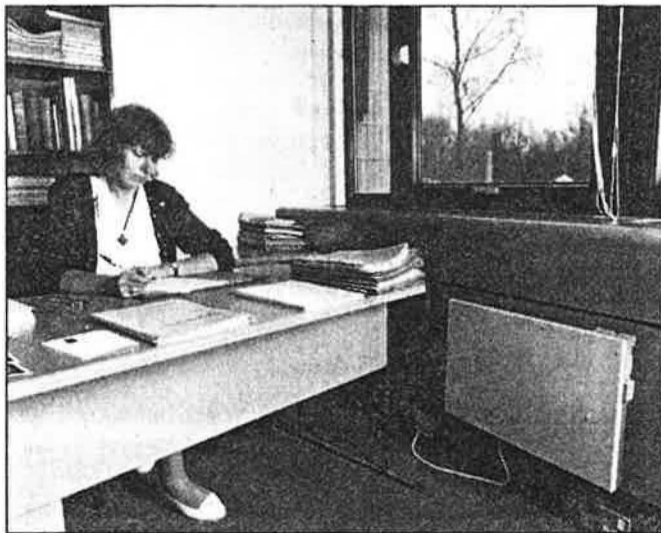
One of the cellular offices with its new electric heater and double glazing.
