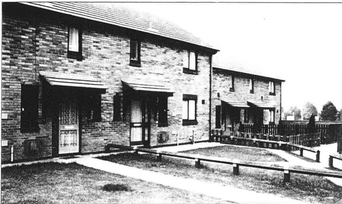
Energy efficient homes at Halliwell Lane Estate, Cheetham Hill, built for Manchester City Council
