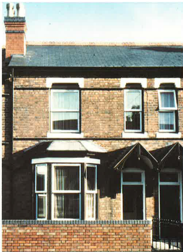
Figure 3 Birmingham enveloping project: house after upgrading
