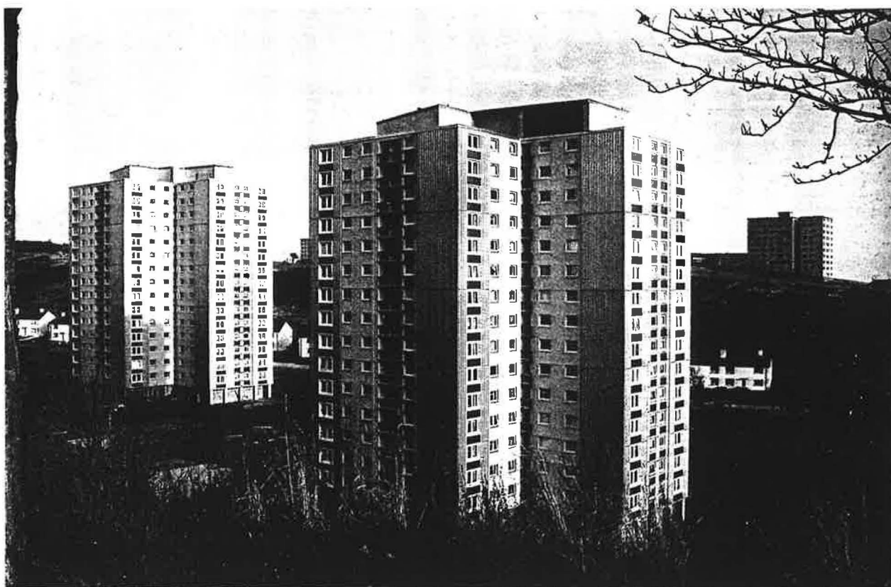
High rise flats, refurbished with external wall insulation, in Greenock, Inverclyde District Council.
