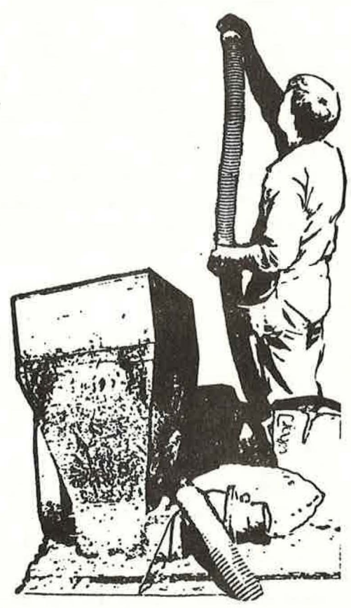
Insulation Blowing Equipment And Installer At Work
