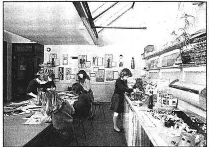
Above: Three south facing lightwells have been set into each classroom wing. The light is channelled down a well to the rear part of classroom and to the toilets.
