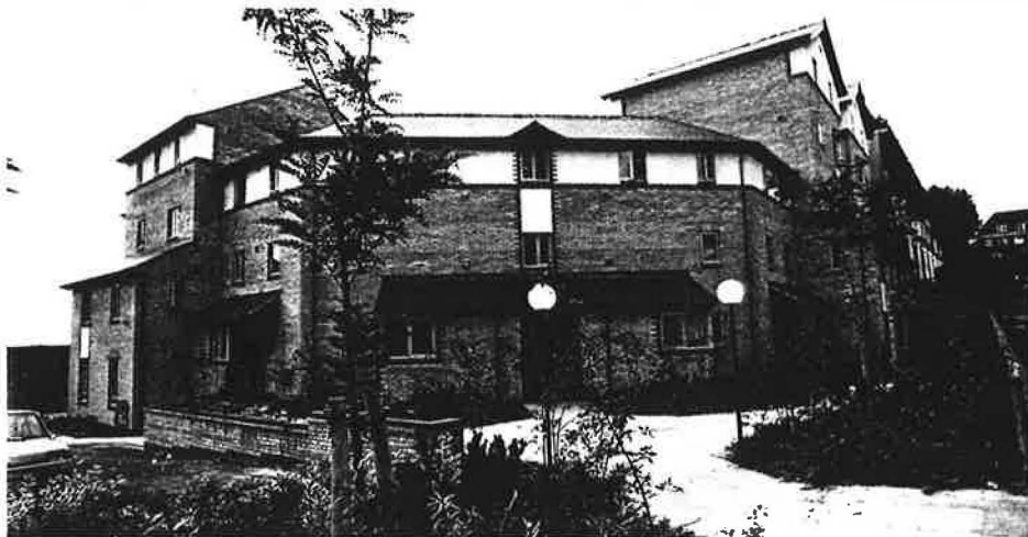
Low-energy flats in Cromartie Road, North London.
