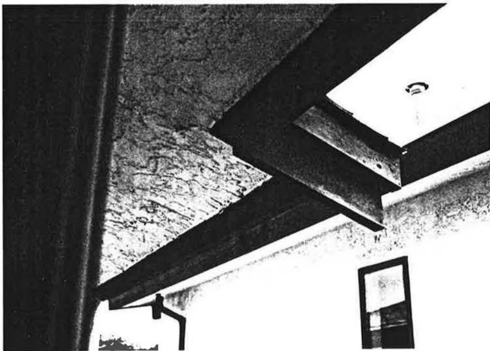
House No.2 - Continuous Soffit Vent
