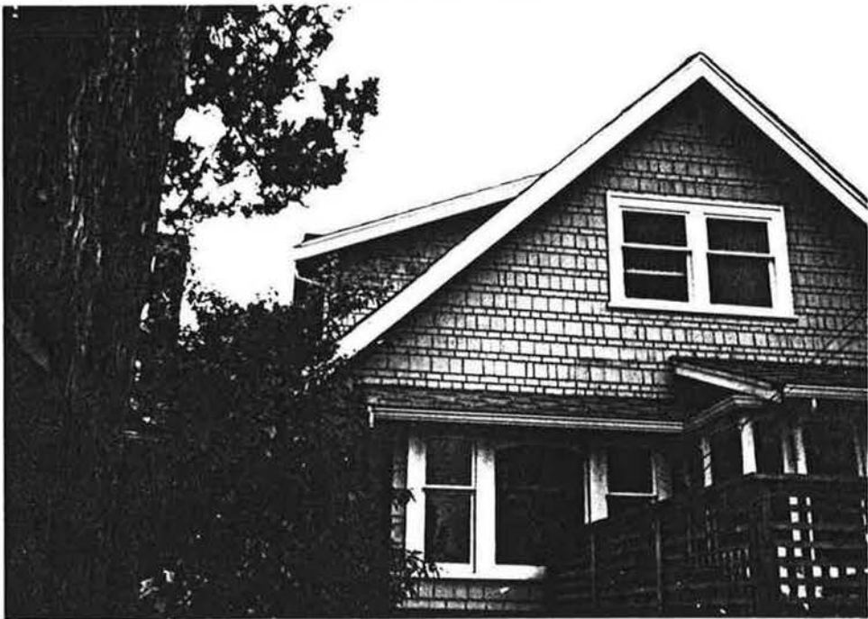
House No.3 - Rear View with Gable Vent and Dormer
