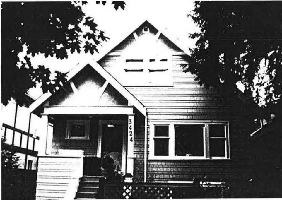
House No.3 - Front View with Gable Vent
